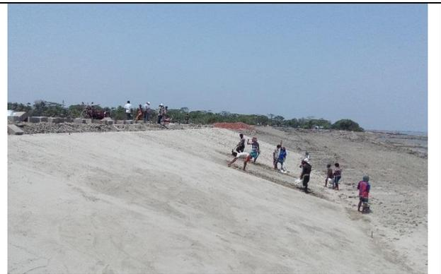
Figure 3-47: Slope protection in Polder-33
