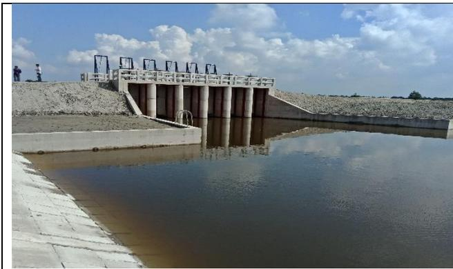
Figure 3-44: Complete of DS 6 Vent in Polder-35/3
